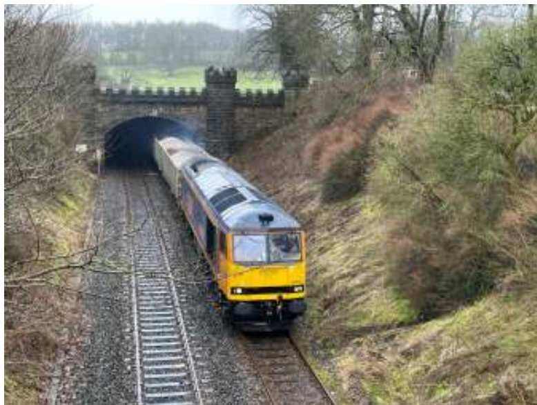
Southbound freight emerging from RVL tunnels
